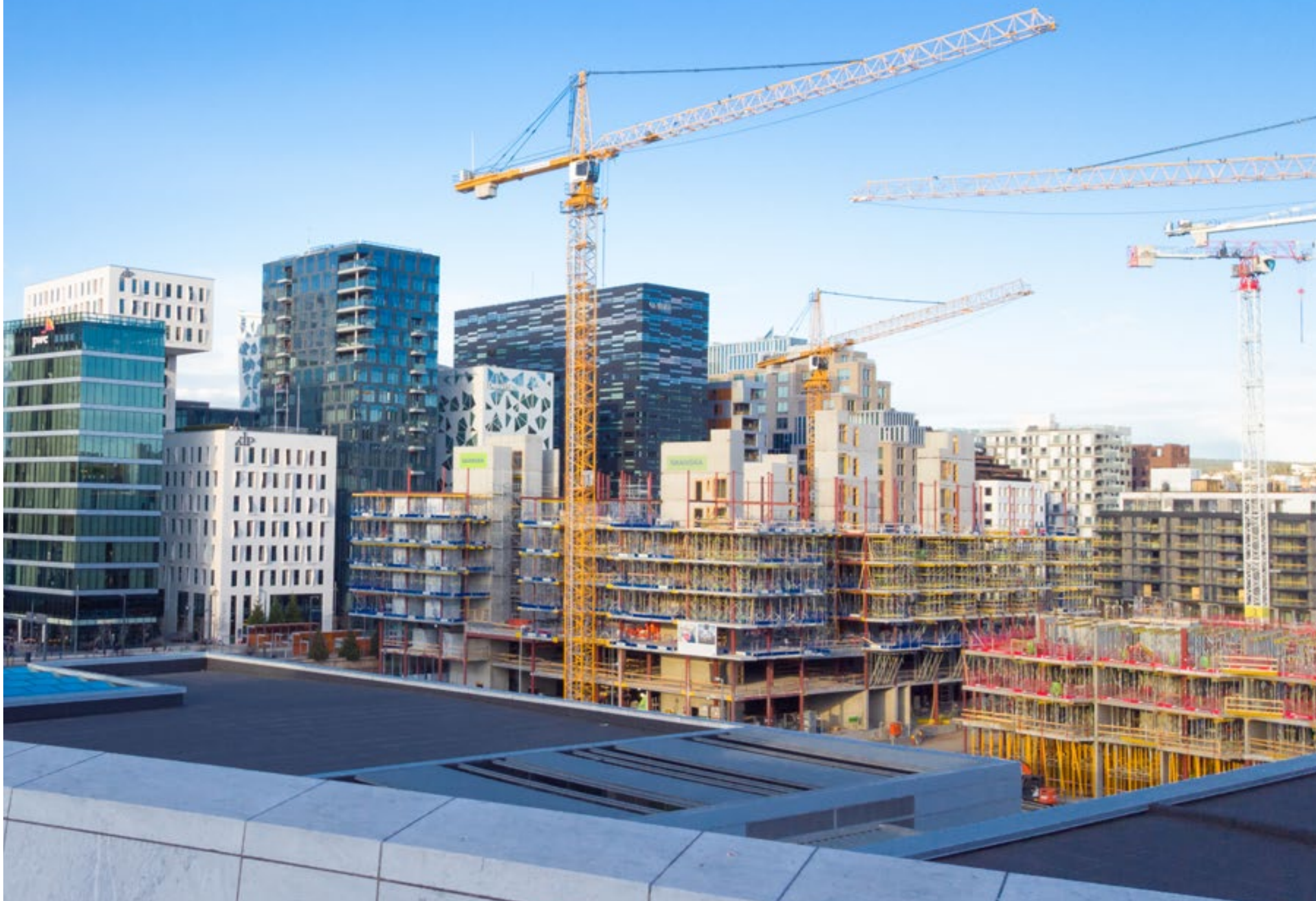
CONSTRUCTION IN OSLO, NORWAY
