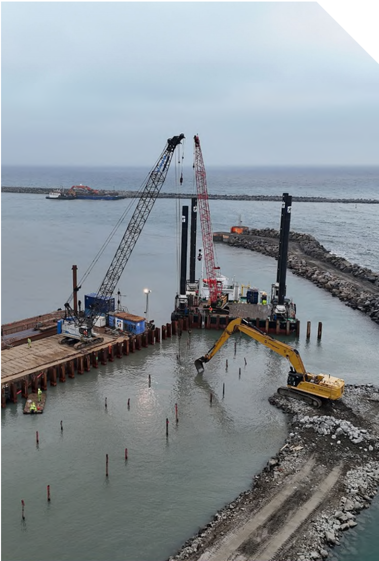
MT Højgaard Danmark’s work at the Port of Rønne is progressing according to plan. The photo shows personnel and machinery carrying out anchoring work. The project will be handed over at the end of the year.
